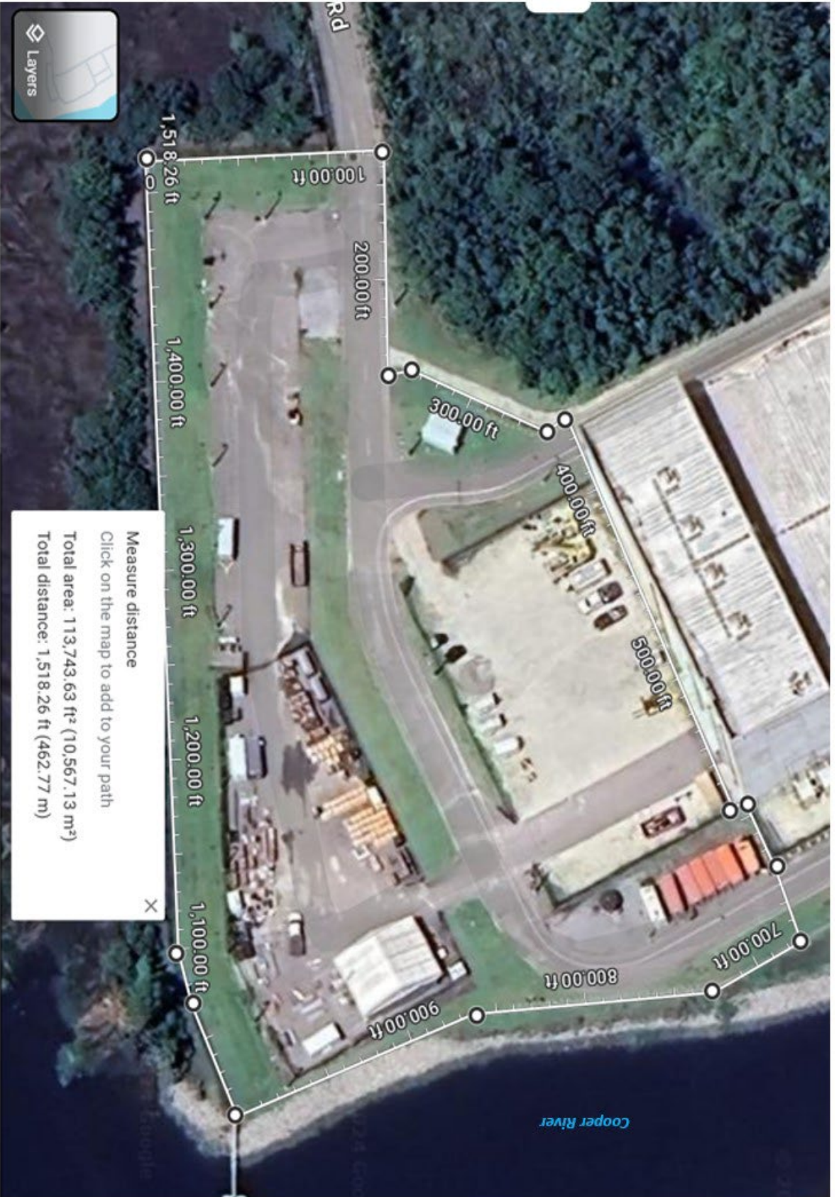
Figure 3: Aerial View of Construction Area
